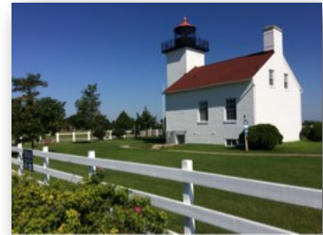
Sand Point Lighthouse in Escanaba.
