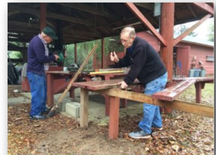
Jim Johnson and Ron Cherry repair the cook shed table.
